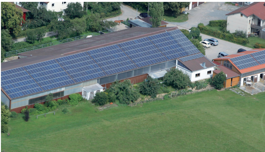
Gäufelden-Nebringen - Germany System: 31,85 kW | SpeedRail
