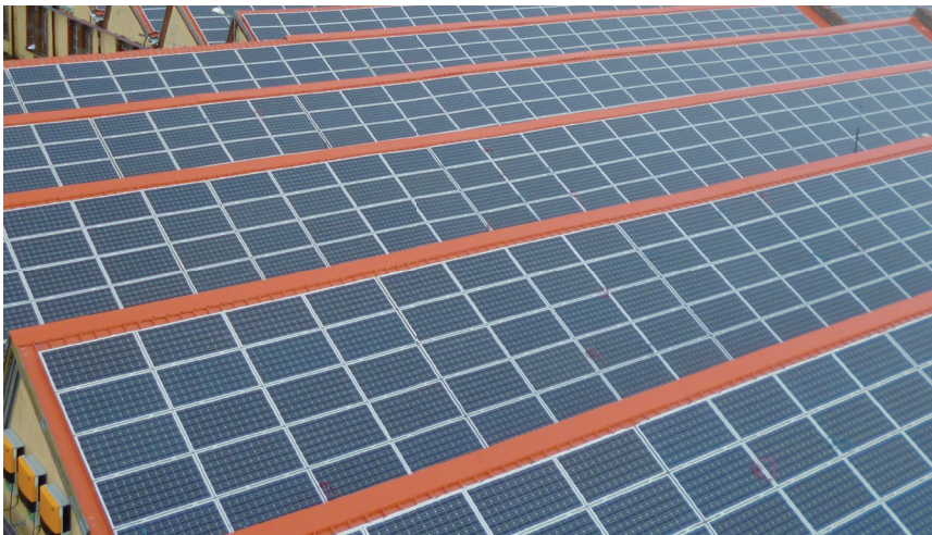
Cernay - France System: 1,136 MW | SpeedRail with AddOn
